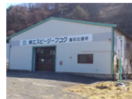
Kamaishi branch office
