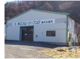
Kamaishi branch office
